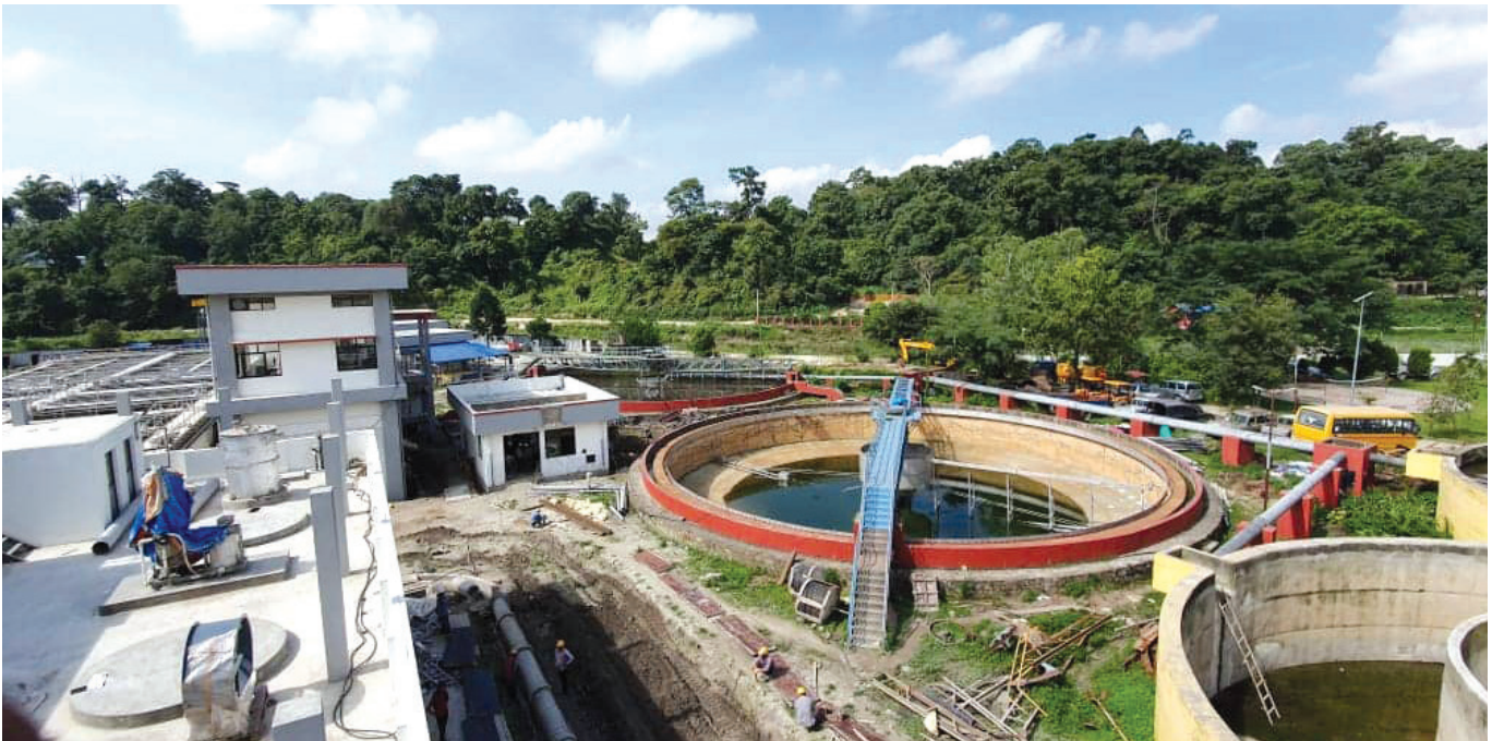
■ A view of the modern, environment-friendly wastewater treatment plant (WWTP) that is under construction at Guheshwori, along with the existing WWTP.
