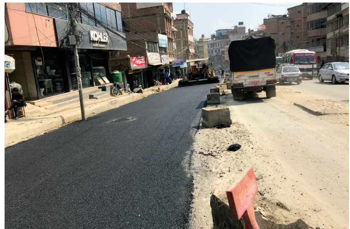
■ Road reinstatement underway after installation of water supply pipeline at Teku, Kathmandu, on May 3, 2019.
